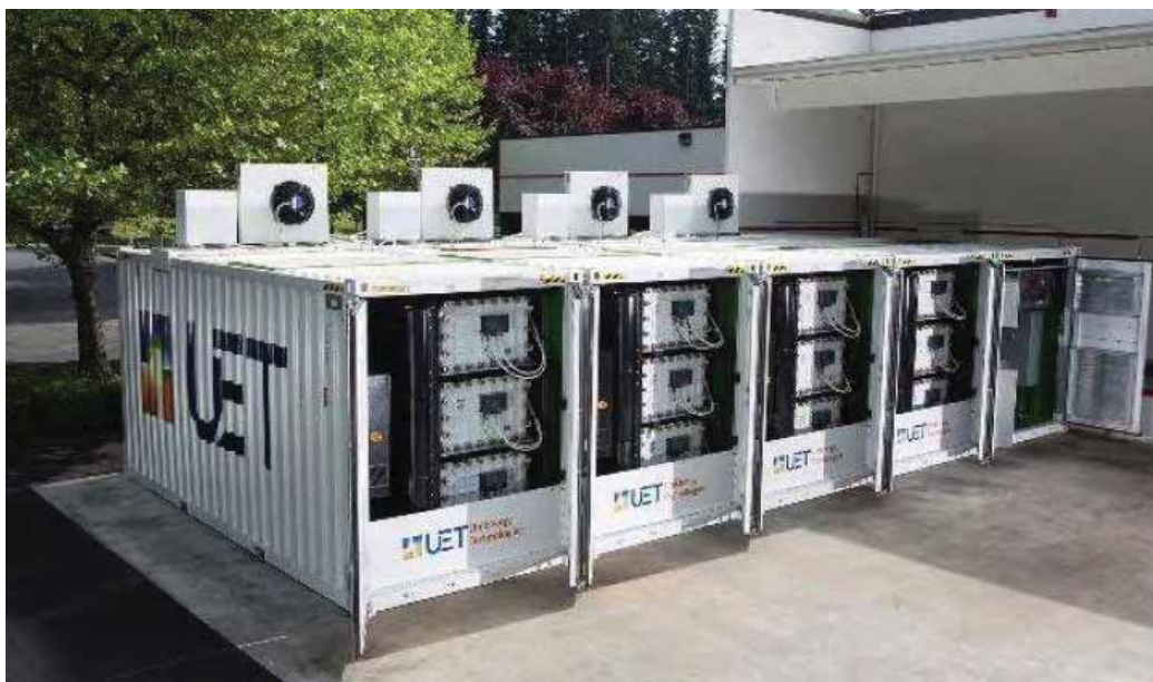
Vanadium redox flow battery storage
