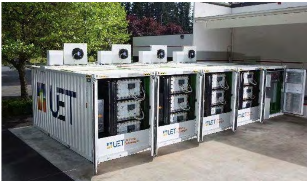
Vanadium redox flow battery storage
