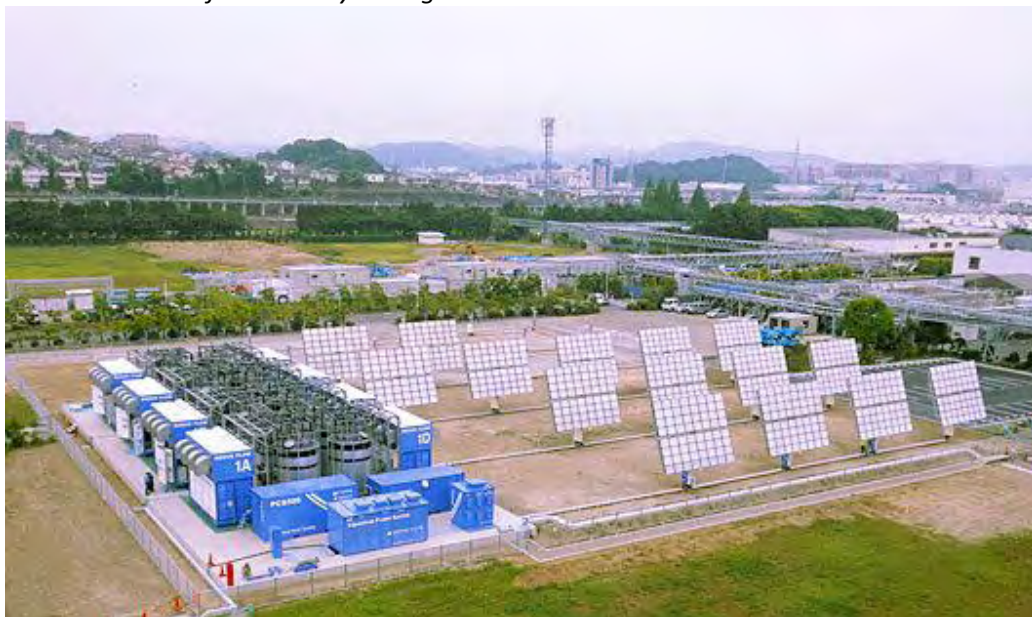
Vanadium redox flow battery storage
